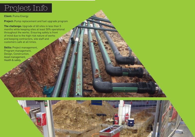
Looking to breath new life into an existing network, the upgrade works on each site required a significant change to the UPSS. Over a 4 week period per site, Switch in conjunction with a number of specialist fuel system contractors upgraded almost all elements of the fuel system
